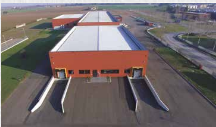
COLLECCHIO - PARMA - PLANT DEDICATED TO HPP TREATMENT
